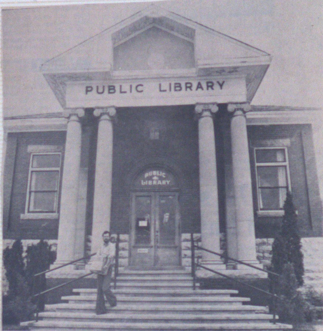
Get ready...get set...move! That's what will be going on towards the end of the summer at the Tillsonburg Public Library, as all of the 18,000 books and pieces of equipment are going to be carted to the Federal Building basement, the home of the TPL while the old library is torn down, and the new library is built. Librarian Matt Scholtz is shown with a box of books, all ready to go across the street, and south on block.
